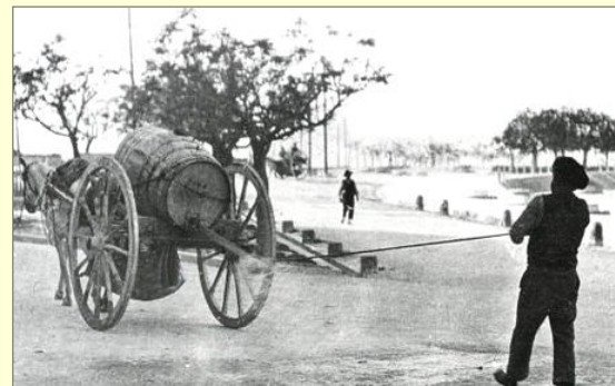
The water-splasher (bexxiex tal-ilma in Maltese) cleaning streets from dust and animal waste which were still mostly unasphalted.
