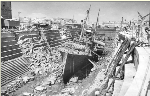
Left: Somerset Dock No. 3 during construction.
